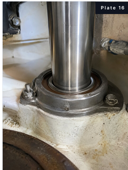
Plate 16. Upper rudder bearing and stock; slight play, monitor (C-3).
