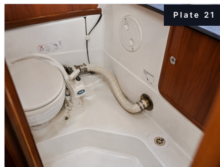
Plate 21. Forward head; sanitation hose permeated and hardened (B-5).
